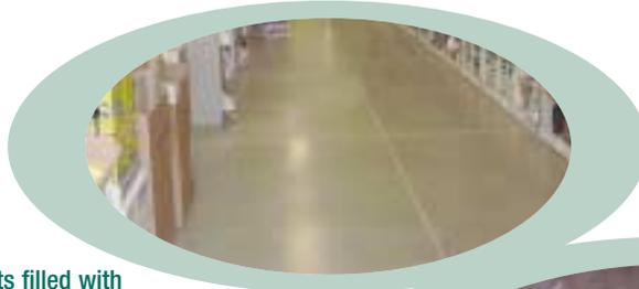
Joints filled with QWIKjoint 200 are well protected from the damaging effects of wheel traffic.
