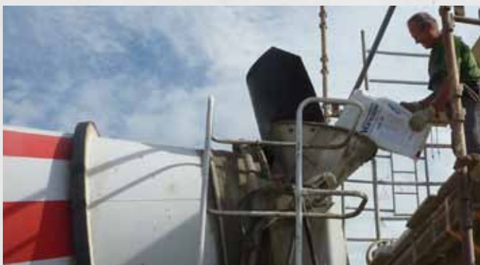
VANDEX AM 10 added at the batching plant.
