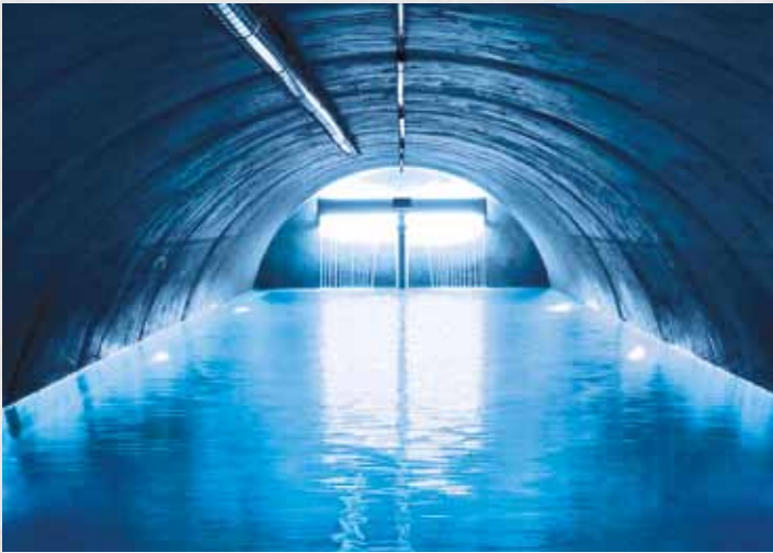
Water containment structures
