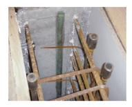
The joint sealant should be applied to a dry, smooth surface. It should be secured with glue and/or steel nails. Where appropriate, the construction joint can also be levelled off using expandable mastic or bentonite paste.
