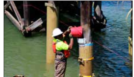
Install 150 mm of FX-70-6MP™ Marine Epoxy Grout to create bottom seal; allow grout to cure overnight.
