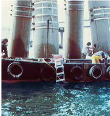
Workboat and divers preparing piling for installation of FX-70® System
