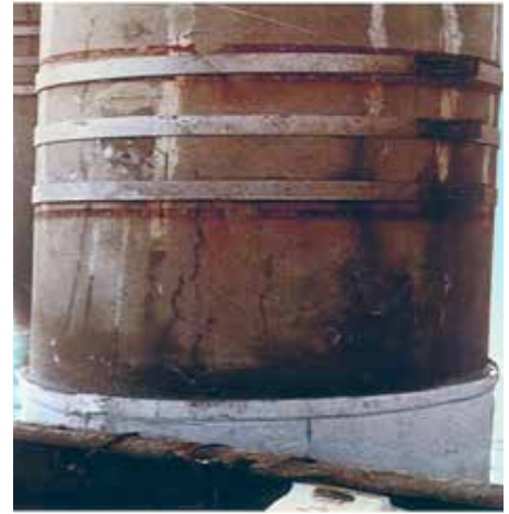
FX-70® System in place and ready for FX-70-6MP™ grout
