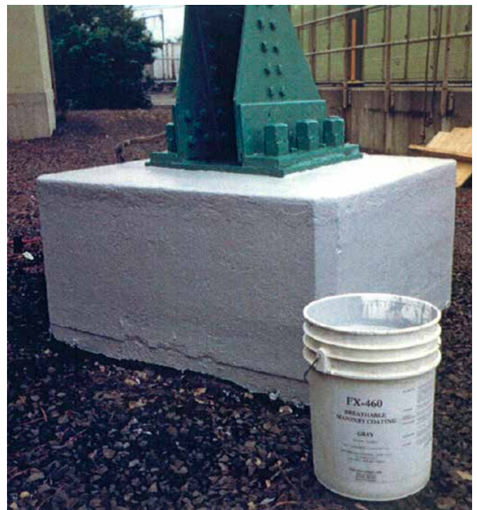
Repair completed with FX-70-6MP™ Multi-Purpose Marine Epoxy Grout as the bottom and top seal material. Coating system is used as a final finish on the outside of the FX-70® jacket.
