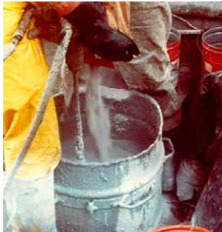
FX-70-6MP™ grout mixed in work boat
