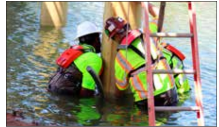
Install temporary bottom seal at base of jacket. Seal may be installed prior to placing jacket.
