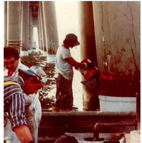
FX-70-6MP™ grout placed in jacket without dewatering
