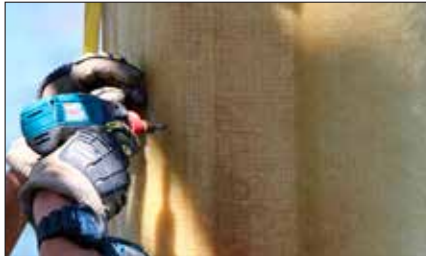
Install a stainless steel, self-tapping machine screw every 150 mm o.c. to secure the tongue-and-groove joint.
