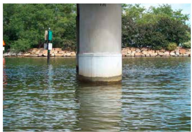
Close-up of a repaired pile
