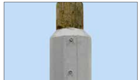
Remove ratchet straps. Repair complete.
