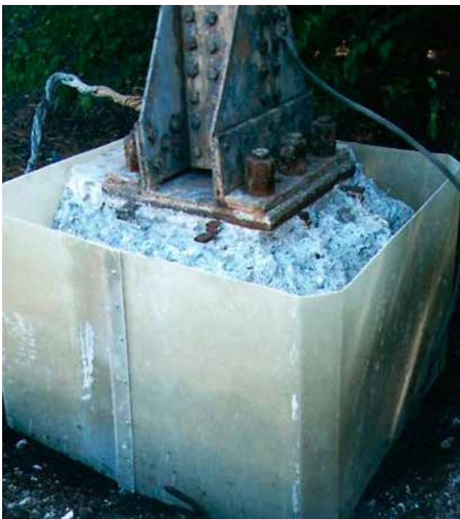
FX-70® jacket installed and backfilled
