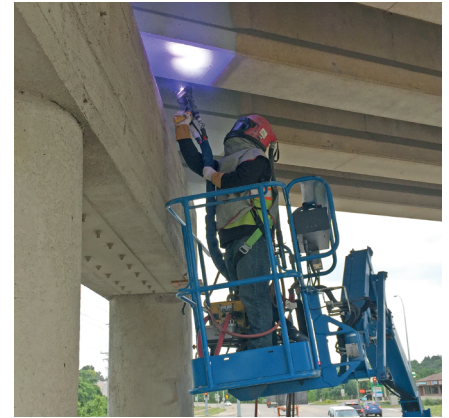
Galvanode® ASZ+ installation
